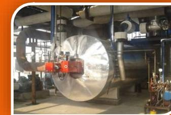
**3.5 MW Thermal Oil Heater for Biscuit Baking**
